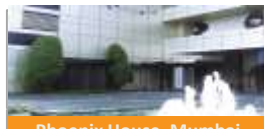
Phoenix House, Mumbai
