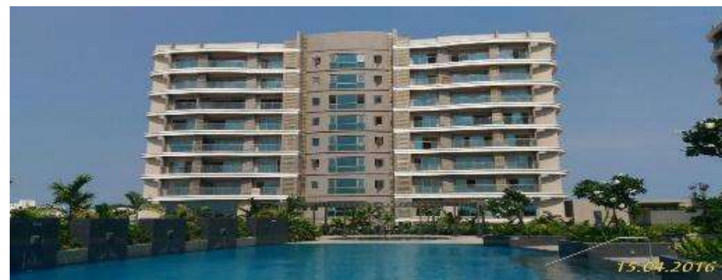
CREST TOWER A
