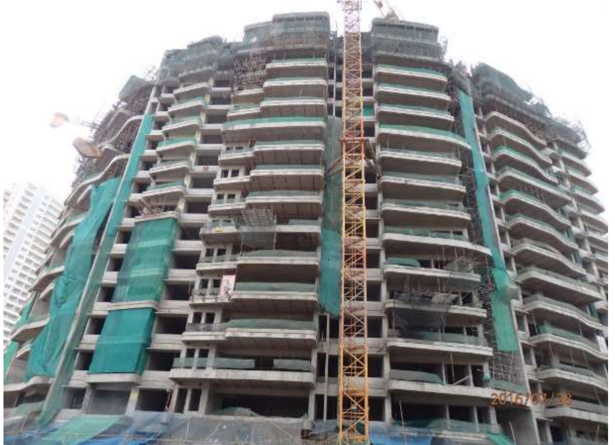
STRUCTURE WORK OF KESSAKU
