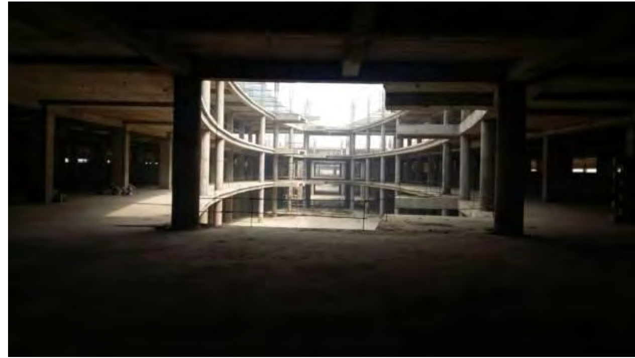
View of Atrium from First floor
