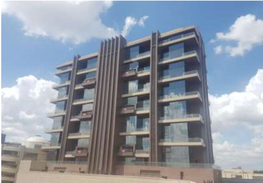
Fountainhead Tower 1 - Front
