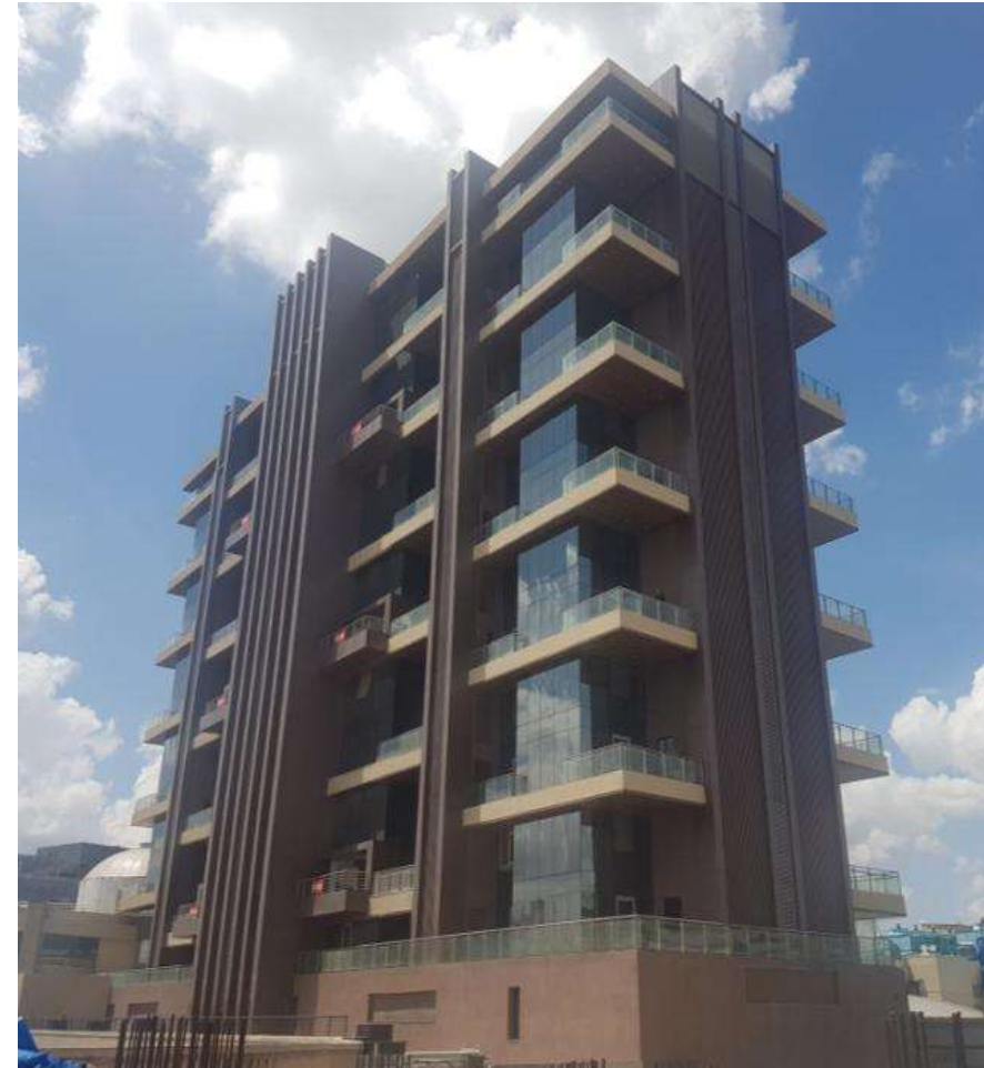
Fountainhead Tower 1 - Side
