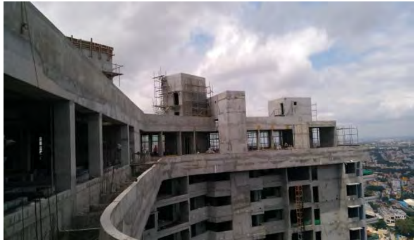
Above Terrace Work in Progress
